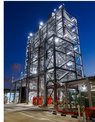
Gradiant's CGE Technology at an industrial wastewater treatment plant in Singapore
